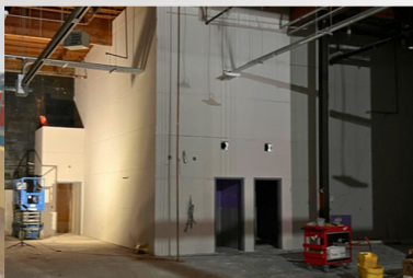
MARCH Drywall & doors completed.
