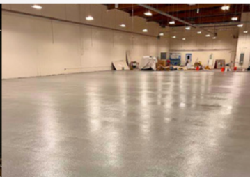
APRIL Paint & flooring completed.
